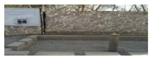
4.**Construction of Percolation Tank with Bore Holes:** A big percolation tank of size 46.5 X 3.5 X 1.5 Meter is made with four numbers of boreholes. Perforations made in the casing inside recharge structure and wrapped with fine net. Excavated pit has been filled with conventional filters.
